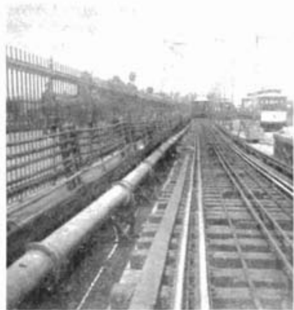
Figure 2 Most mail tubes were buried under the streets, but the Manhattan to Brooklyn tubes crossed the East River over the Brooklyn Bridge. This is the approach to the bridge on the Brooklyn side. (Published in Transactions of the American Society of Mechanical Engineers in 1899)
